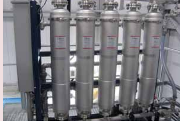
Sand-filter backwash wastewater recycling system using SL modules
